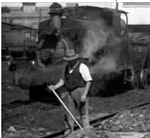
This image was supposedly taken in Lota in 1959, shows a saddle tank loco with a tank commencing at the front tube plate rather than the front of the smokebox. Its identity is unknown.
