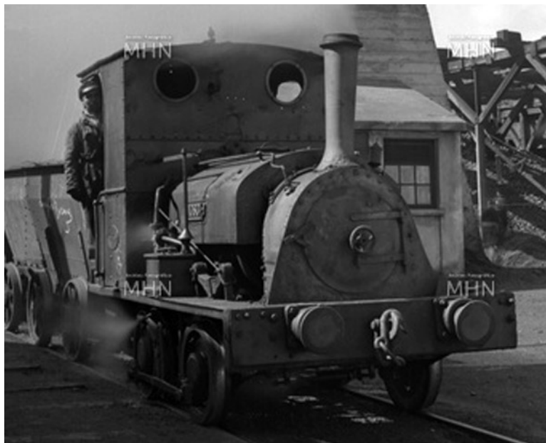
From DIBAM archive at the Biblioteca Nacional, Santiago. The closely-set side buffers were for use with the 'black wagons' as seen behind the loco in this view.
