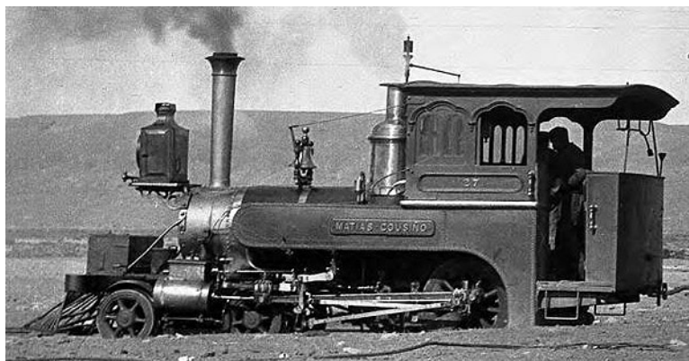
Photo by Dr. Isaiah Bowman 1913, in AGS collection at http://uwm.edu/libraries/agsl/photos/ showing no. 27 at Monte Amarga. Note that the spark-arresting chimney shown in the drawing and photo above has been replaced by a straight stack. The rear bunker is now taller and seemingly more angular than the original, it possibly now being an oil tank.
